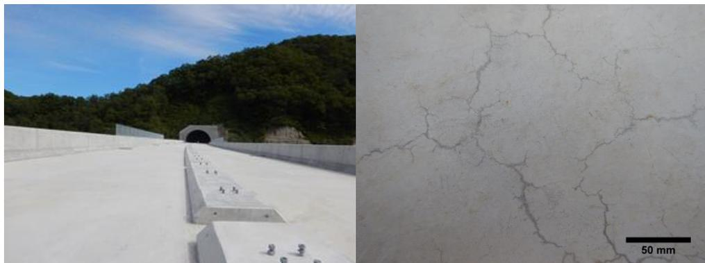
Figure 5.1. Micro-cracks appear on RC bridge slab.
