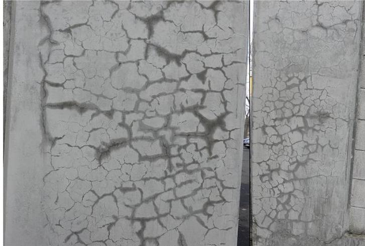
Figure 1.4. Early-age shrinkage cracking of RC structures.
