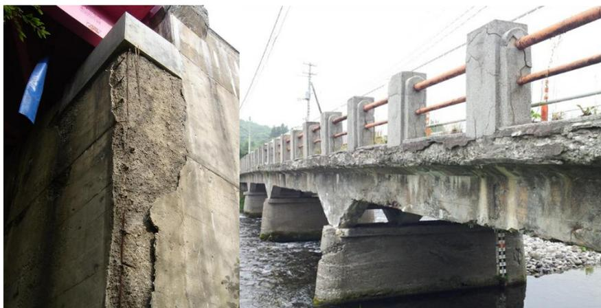
Figure 1.2. Deteriorated RC bridge structures (Mainly frost damage).
